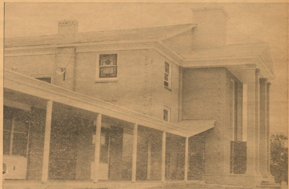
Summer saw the First Baptist Church complete their $50,000 remodeling project. This view shows new educational annex and new glassed-in porch.
