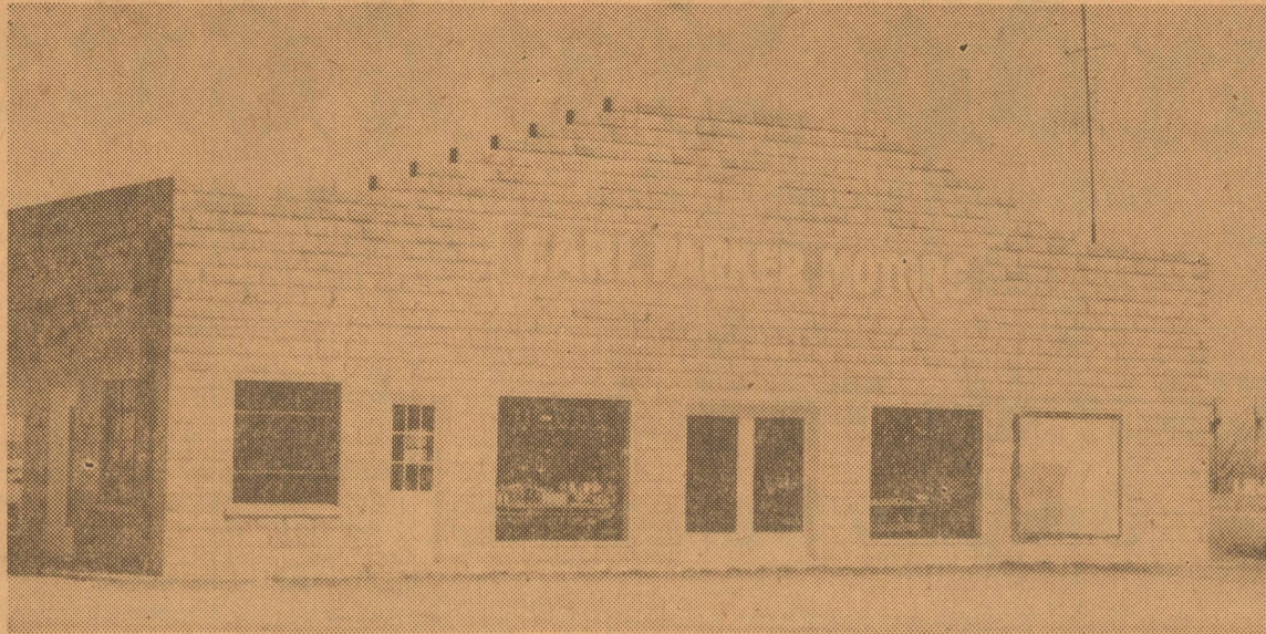
From This— Building was a familiar sight last generation
