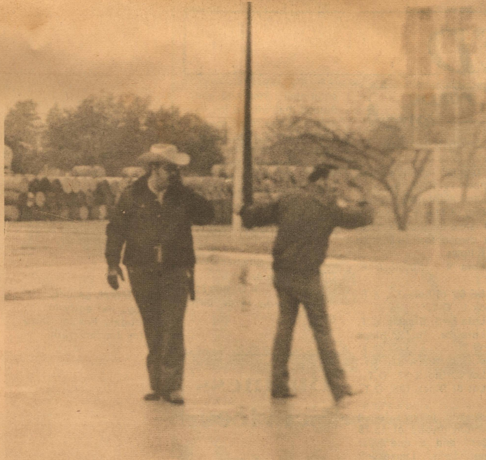
Last Friday hand signals from Sheriff's deputies helped control the traffic during the power failure. The electricity was knocked out temporarily because of a transformer fire.
