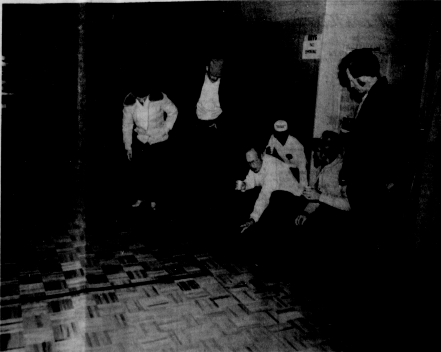
SCHOOL BOARD MEMBERS met at 7:30 Monday morning to inspect the remodeling job at the McLean school gymnasium. The board postponed accepting the job until Thursday morning
