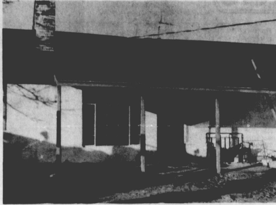
Pictured is the home of Mr. and Mrs. Johnny Carpenter following a fire Sunday which totally destroyed the structure and contents. (Photo by Linda Haynes)
