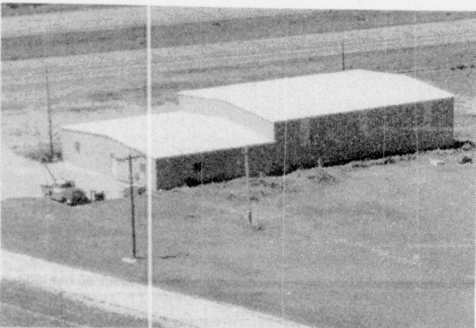
Britten Supply's present home built in 1978. It is conveniently located just south of the Britten home, one mile west of Groom.
