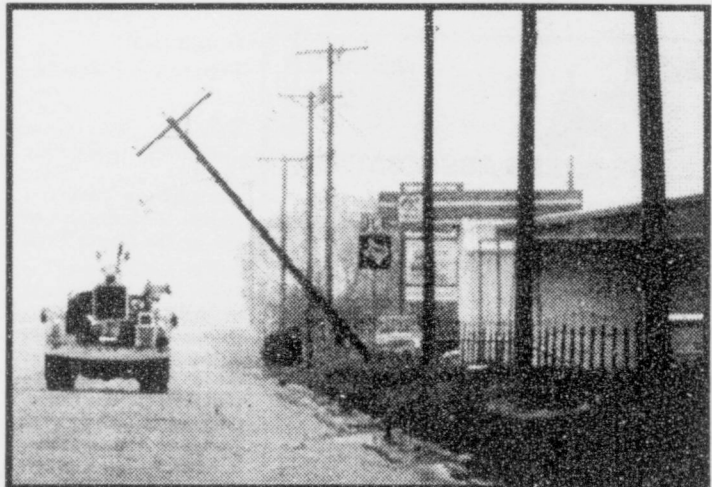
Spring storms have made their appearance in the City with about 1.5 to 1.75 inches of rain following in the last couple of days. The soggy ground gave way and this light pole is definitely needing some help!
