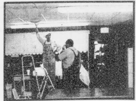
Boots Stone & Dan Eggers make repairs on ceiling.
