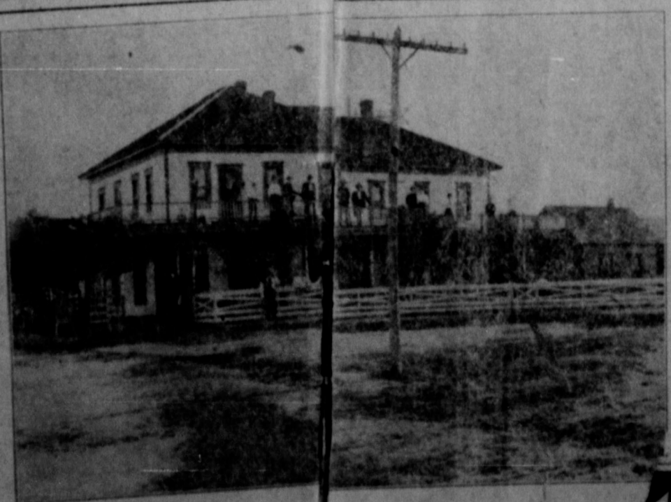
One of Our Civic Buildings—Hotel Hindman
