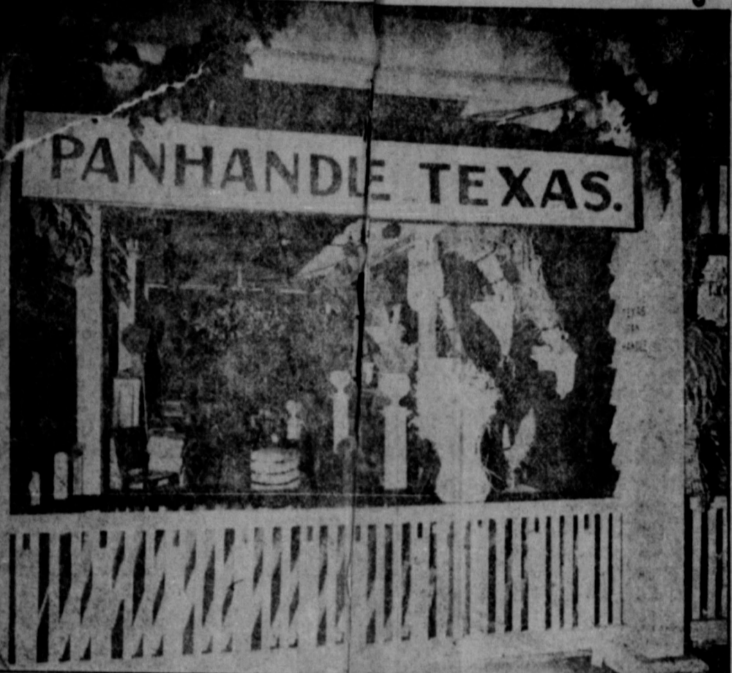
Interior view of Panhandle Exhibit at Recent Land Show in Chicago
