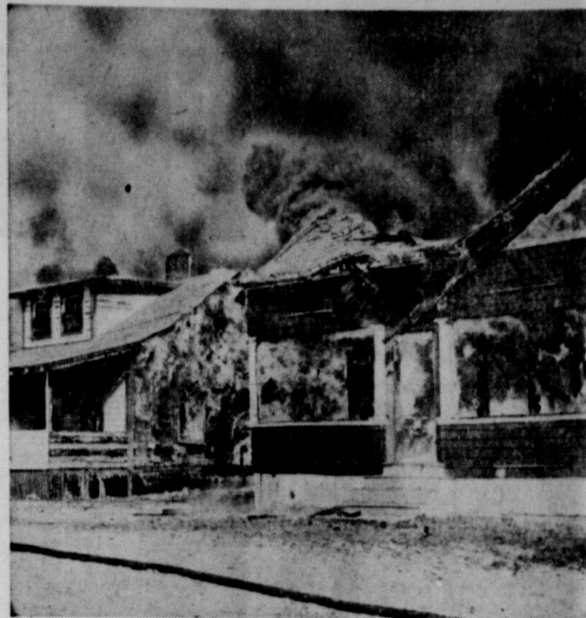
Damage estimated at about $2,000,000 was caused in the Ocean Bluffs, Mass., area as the result of a fire that destroyed a church and leveled more than 450 cottages. Only a timely shift in wind saved hundreds of other houses. The above photo shows a row of cottages burning fiercely when the fire was at its height.
