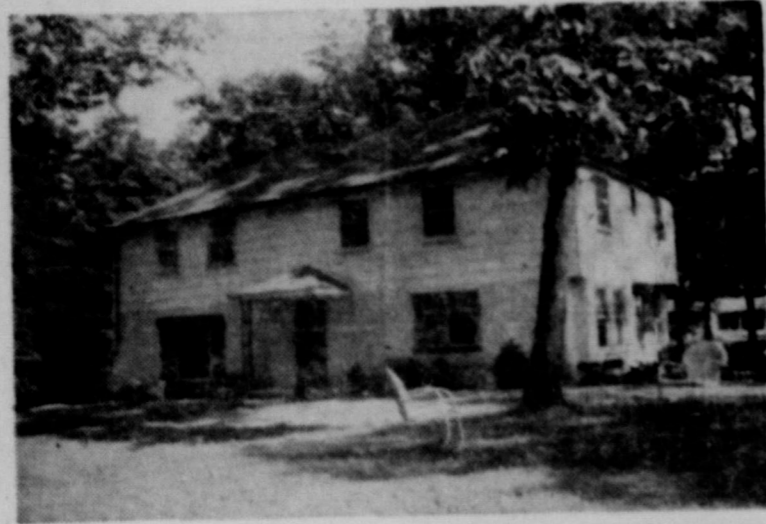
Concrete, asbestos and asphalt provide economical, fire-safe construction in this home expansion project. The new roof of asphalt shingles in a green blend provides color contrast with the white sidewalls.
