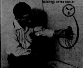
"This is the wiring for the electric dryer as it appears before the three-wire outlet is installed and the walls finished. It's easier to get the right wiring at the time the house is being built. I've planned mine accordingly."
