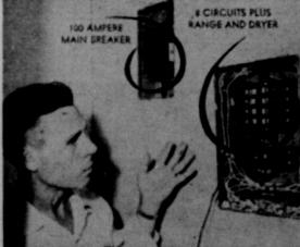
Here you see 8 circuits with provision for a future 8 more. In addition, there are separate circuits for the electric range and electric dryer. The kitchen, for example, has two appliance circuits for coffee-makers, waffle irons, toasters, etc."
