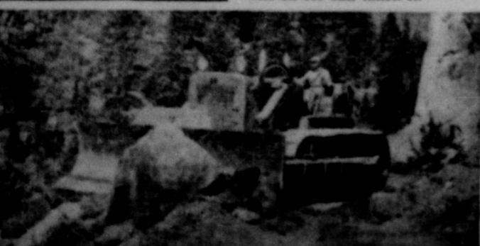
READY FOR TOURISTS —Twisting road up Colorado's famed Pikes Peak is graded by International TD-24 crawler tractor for summer flood of tourists. About 250,000 people a year drive to the 14,110-foot summit and there has never been a serious accident since the road was built in 1914.
