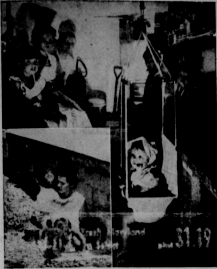
HARRY E. THOMASON , his wife and five children gather in the bomb shelter he built for $350 in his spare time at his home at District Heights, Md., eight miles from downtown Washington. Top of shelter doubles as front porch. Mrs. Thomason is shown (inset) emerging from the escape hatch, which would be filled with sand during an attack to keep out radioactive dust. The shelter includes a tunnel entrance to basement, an electric or battery-operated air blower, running water, a fire extinguisher, plenty of food and basic tools. (Washington Star Photos)
