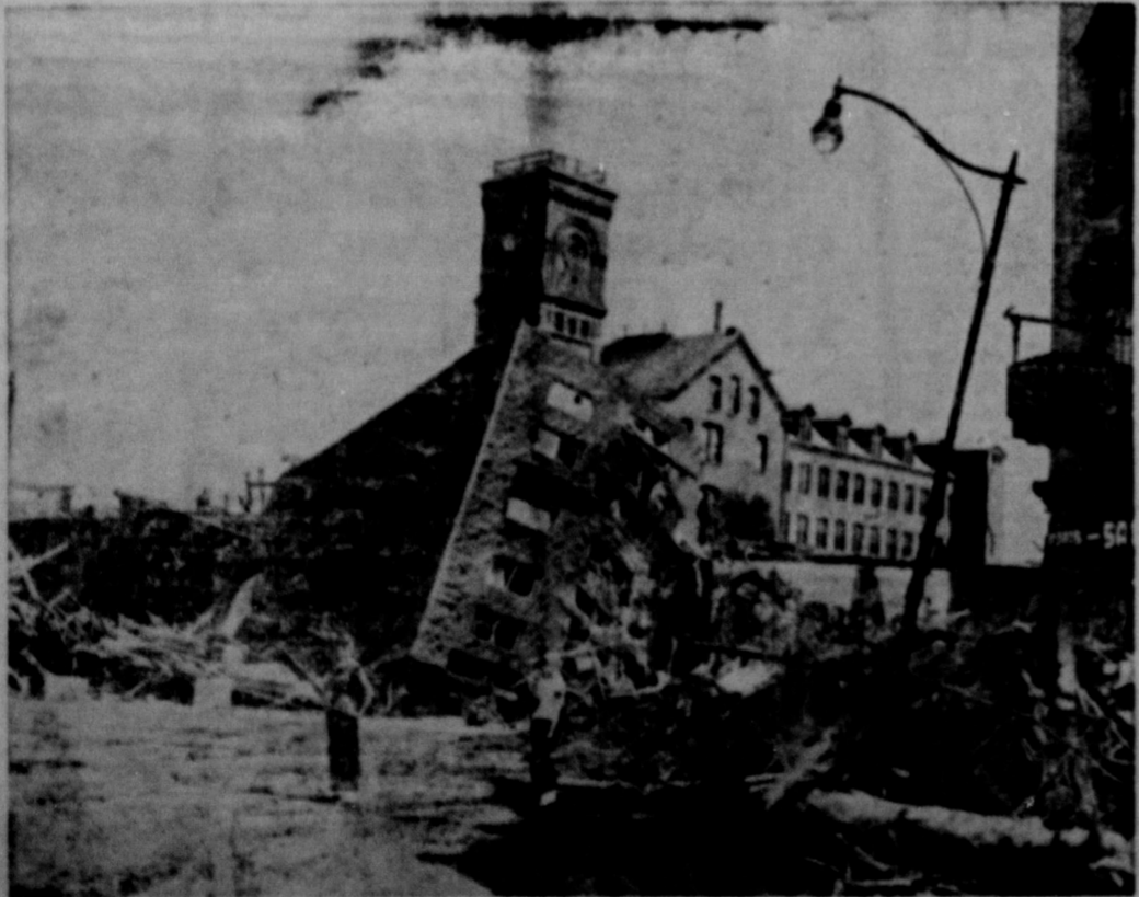
CRUSHED AND BROKEN, this 16-family apartment house in Waterbury, Conn., was left high and dry after the rampaging Naugatuck River receded August 21. This was a sample of devastation in the flood which, according to the Red Cross, destroyed 1,236 houses and badly damaged 6,988.
