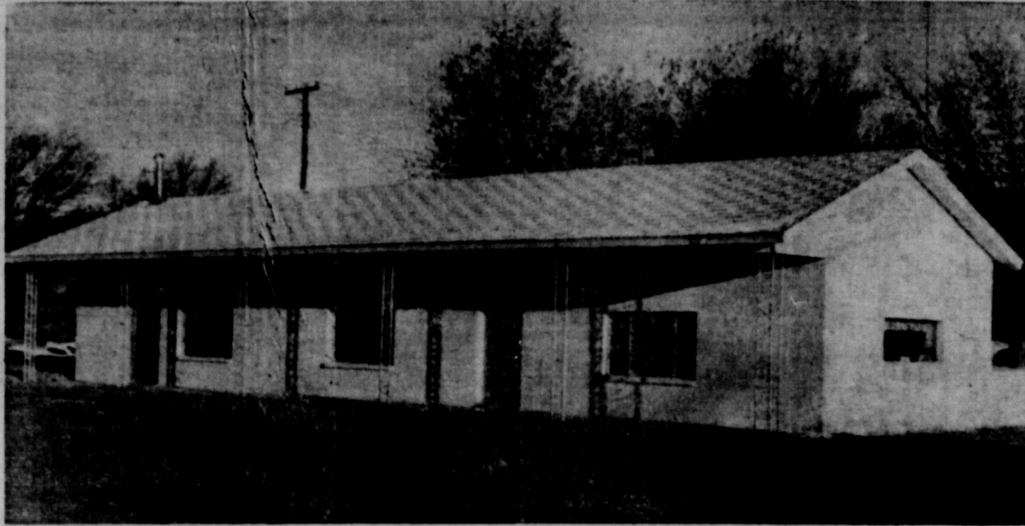
THE FIRST BAPTIST CHURCH will observe open house in this new nursery building Sunday afternoon from 3:30 to 5:00 o'clock. The air conditioned building will accommodate 50 children and has a fenced play yard.
