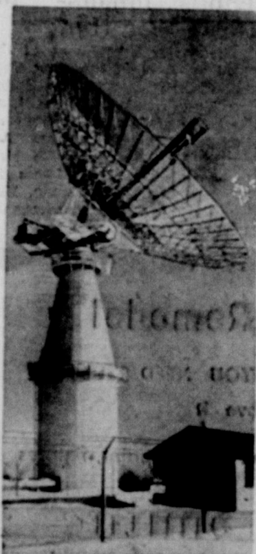
SNOOPING ON VENUS —History-making first contacts with any celestial body beyond the moon was made with the radar pictured, above. The two electronic contacts with Venus were made in February of 1958, and only recently revealed. Signals broadcast from Massachusetts Institute of Technology's Lincoln Laboratory at Westford, Mass., made the 56-million-mile round trip. Months were required to sift the sounds from a jumble of recorded space static, and to make certain that the signals were, in truth, received.
