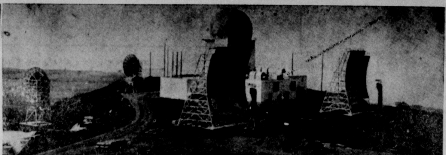
OUT OF THIS WORLD —Other-worldly look of the structures, above, fit the bleak site on which they're located. On Unimak Island, far out in the Aleutian chain, the group of buildings are part of the westernmost link of the transcontinental DEW—Distant Early Warning—network. Churchlike dome, center, houses radar unit. "Dishes," left, and curved reflectors, right, are portions of radar detection and beam-casting communications equipment.
