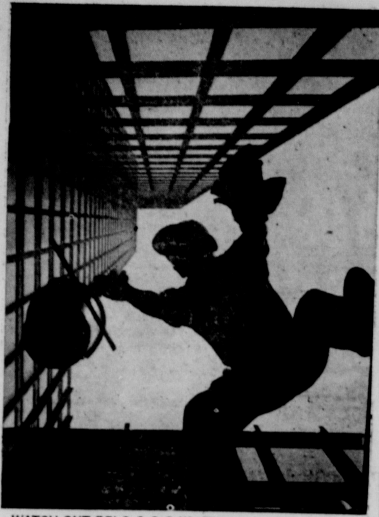
WATCH OUT BELO-O-O-W—Enough to make one cringe away from the picture is the sight of Oxy Paraszczak, hurtling toward you down the side of this building. He's perfectly safe, atop glass canopy on lower level of a New York skyscraper.
