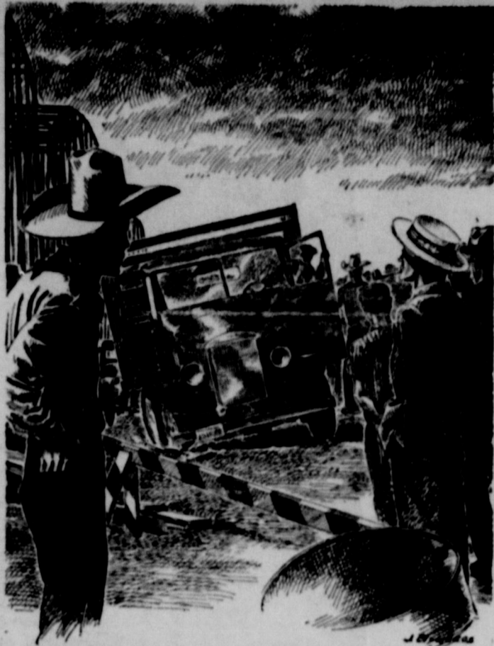
Will Wilson explains that the "Bridge War" between Texas and Oklahoma concerned the opening of three free bridges across the Red River. "Crossing the Gainesville bridge a large truck found the Texas side impassable."
