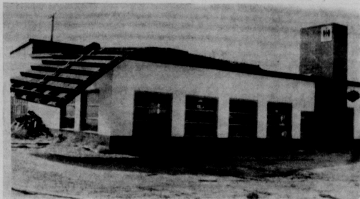
ROOF SHEARED BY WIND—Pictured above is Andrews Equipment Company building following the strong wind that lashed the area Tuesday. A section of the roof of the building was torn loose and thrown across the end of the structure. Damages over the community from the high winds ran into several thousand dollars.
