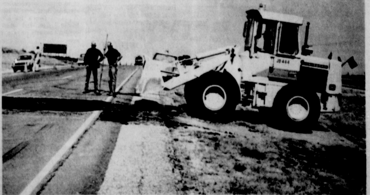
THE HIGH TEMPERATURES in McLean have been dealing the state highway maintenance crews misery. Here, men repair a section of I-40 east of McLean which exploded because of the heat. (Photo by Linda Haynes)
