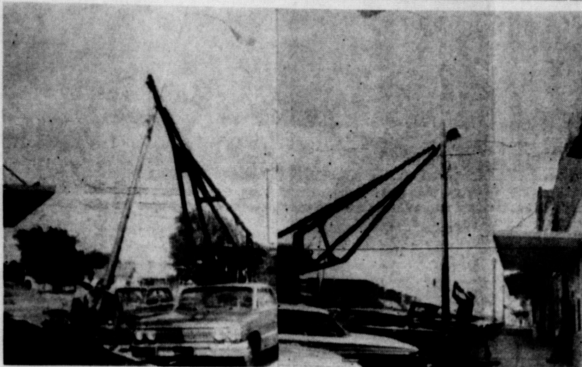
LIGHTS GOING UP! — Southwestern Public Service has completed the 1st phase of installing mercury vapor lights in McLean. These new lights are set 30 feet high and provide more than twice the light of the old street lights.
