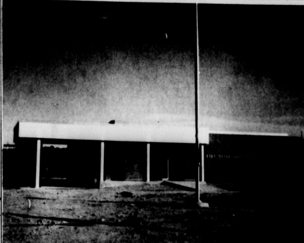
READY FOR OCCUPANCY --With only some finishing touches to be added, this new division communications headquarters for the Texas Department of Public Safety is ready for use by Department personnel. On a 200x200 foot lot, the building will provide offices for all DPS field service personnel in the area, including the Highway Patrol, Driver License and Weights Division, Motor Vehicle Inspection Division, Texas Rangers, plus the radio communications crew. At least five new families will be brought to Ozona as a result of establishment of the communications center here. Antennas for the DPS radio will be mounted on the 500-foot tower located at Crockett Heights, five miles east of Ozona.
