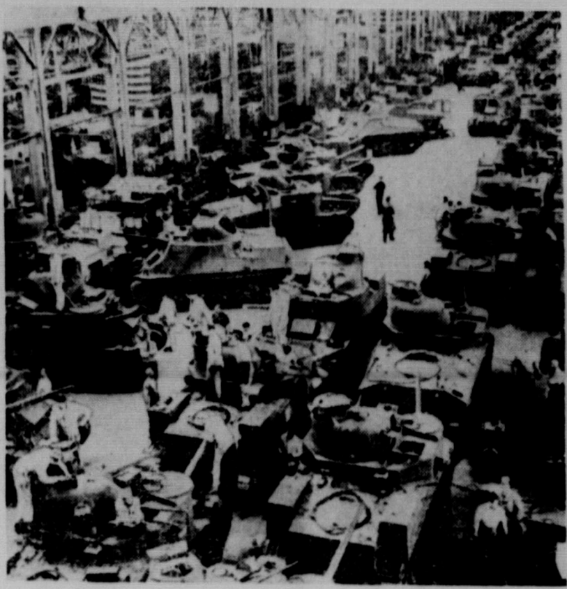
This is a view of the Chrysler plant in Detroit turning out land battle-ships by the hundred. Imposing as it is, this is just a cog in the mighty machine now in high gear turning out the sinews of war to defeat the Axis. Production has now hit its stride and the tanks roll off, night and day, in a steady stream.
