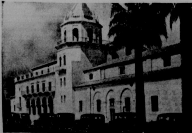
Here, beautifully situated amid palms, is the new municipal auditorium in San Jose, Calif. It was erected with the aid of a PWA grant of $500,000, and is the first unit of the city's proposed civic center.
