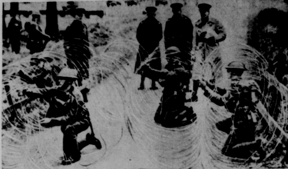
English troops shown at work interlocking coils of steel wire tough enough to stop light tanks and armored cars during a demonstration of modern infantry equipment at Mytchett, Aldershot. Tests of the equipment by the South Staffordshire regiment indicated that it has practical value.
