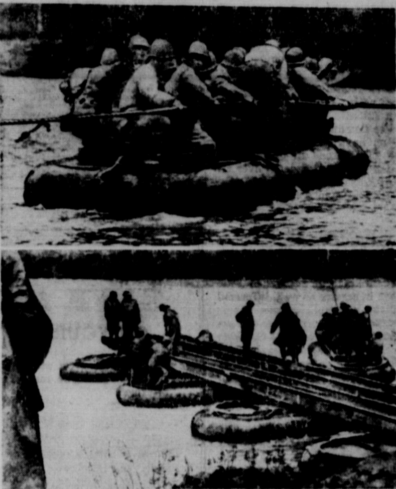
Despite strong German defensive action, Allied forces pushed across the Voltorno river in their steady northward march over Italy. Top: American infantry troops tow themselves across the strategic river on a rubber pontoon. Bottom: A group of American soldiers pitch a steel pontoon bridge across the Voltorno while a sentinel guards against snipers.
