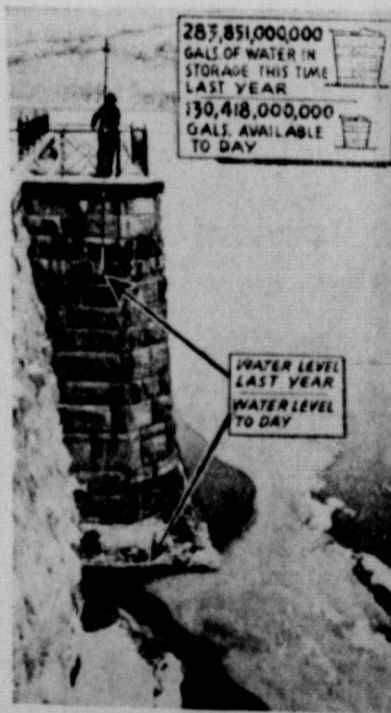
Photo-diagram shows the seriousness of New York city's water shortage, due to last year's drought. The reserve water is only 46 per cent of the 1939 total at Croton reservoir. Gatehouse Foreman John Tompkins indicates with a pole the point to which water usually reaches.
