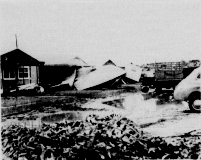
NEW TEACHER homes, just completed, took a beating from the flood. A trailer house, center background, roof and all manner of debris crashed into the new cottages but none was washed away.
