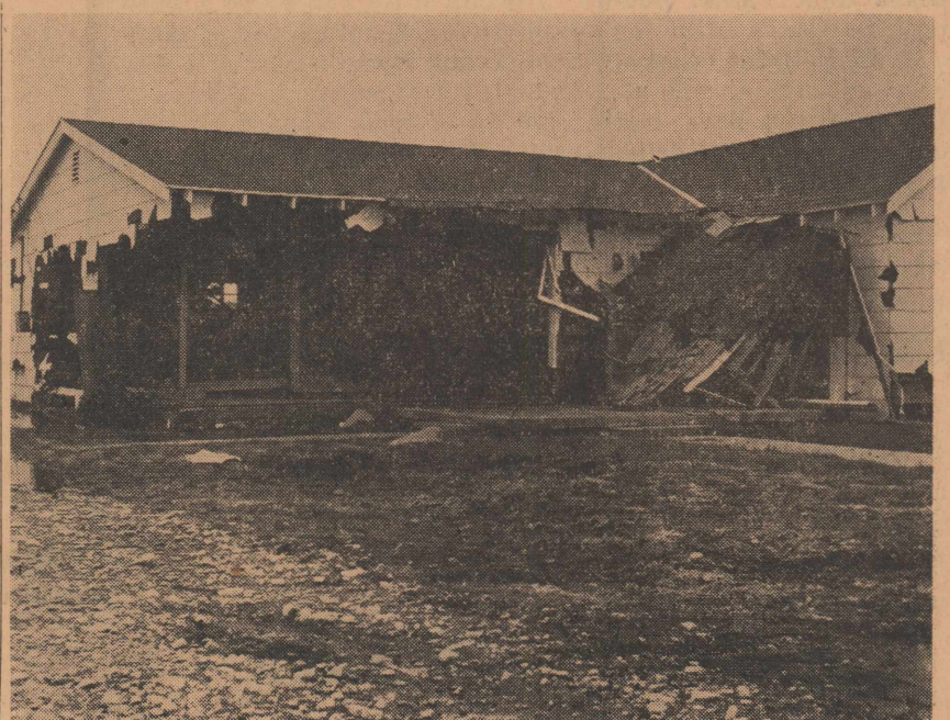
DESTRUCTIVE FORCE of the flood water is illustrated in this picture of the Joe Friend home. Floating houses, garages and other objects crashed into other homes, either dislodging or wrecking them.
