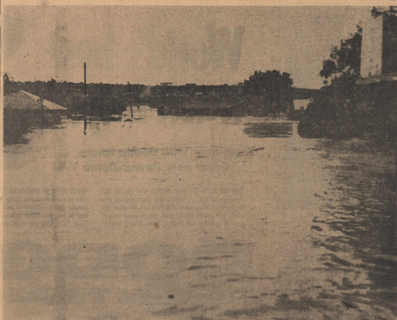
RUSHING WATER climbed high on Ozona homes in its mad rush as it spreads from hill to hill to cause millions in property damage and to take fifteen lives. The above scene pictures the C. W. Taliaferro rock home withstanding the onrushing water.
