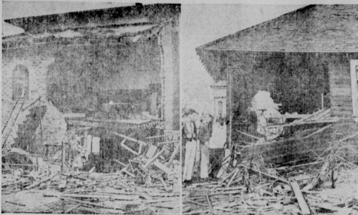
Death was cheated by one hour's time recently when a water heater exploded in the Ripon junior high school at Modesto, Calif. The heater blew up at 6:55 in the morning and ripped out a whole corner of the athletic building, left. It sailed 150 feet through the air and was projected through the agricultural building, right, piercing both walls of the structure like a giant cannon ball.
