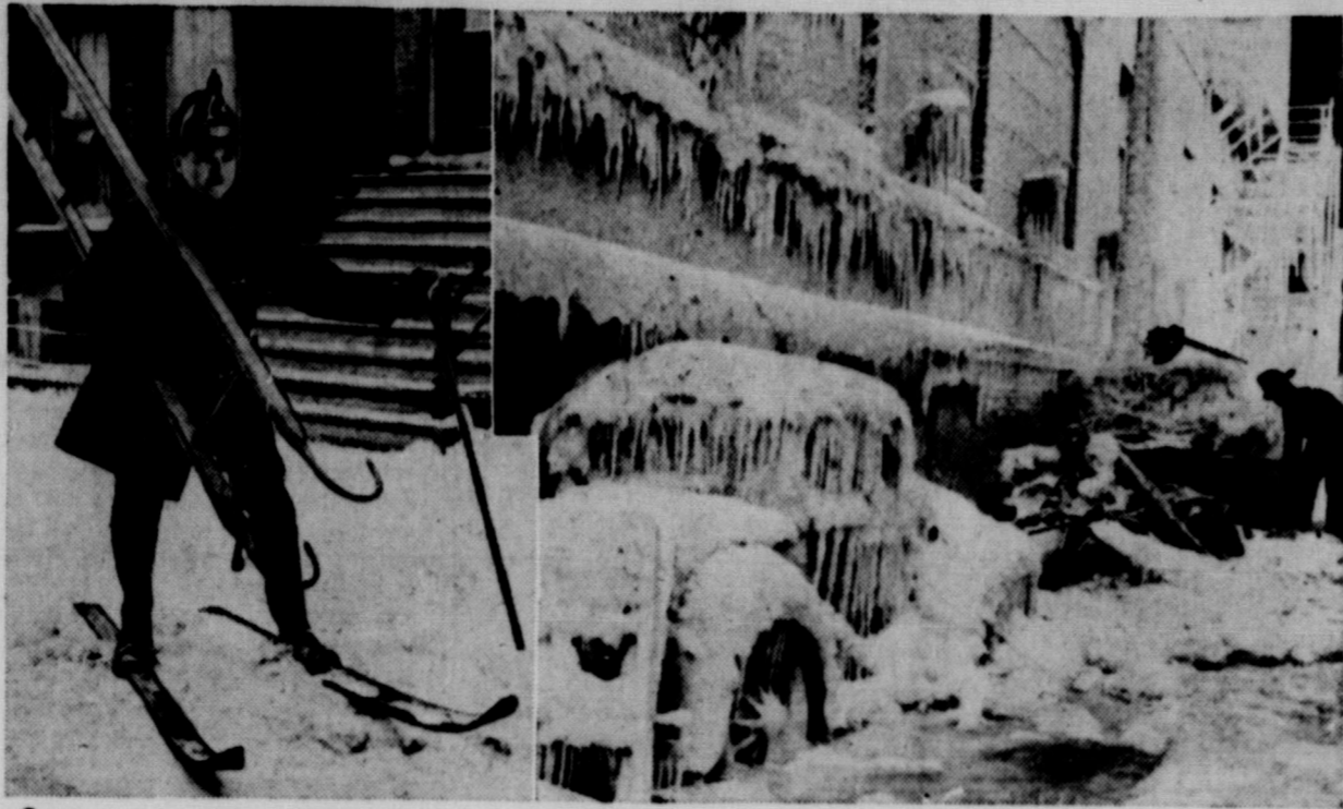
Subzero weather in Chicago proved a dangerous handicap to Windy City fire fighters recently. Heavy snow and freezing temperatures called for drastic measures. Firemen John Donovan, left, equipped with skis and carrying a ladder, hastens to a fire just outside the city's Loop. Right: A parked automobile sealed with a heavy coating of ice from water sprayed by firehose. After each blaze firemen were forced to chop their hoses free from ice-covered streets.
