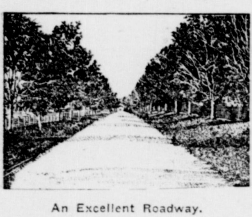
An Excellent Roadway.
