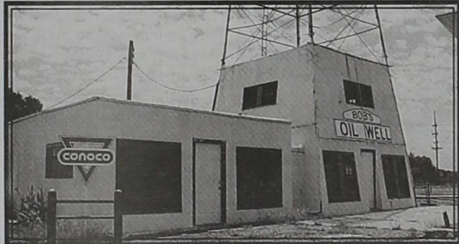
NOW: Renovated through citizen volunteerism and private donations in 2004, the historic site has completed Phase I of its intended repair.
