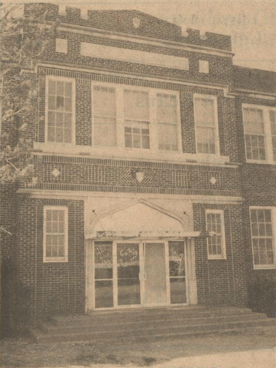
OLD SCHOOL HOUSE -- The fate of the former Matador High School building is resting in the hands of the Motley County School Board. A group of citizens is trying to save the building which may be torn down to make room for a parking lot. (Photo by Leon Watson)
