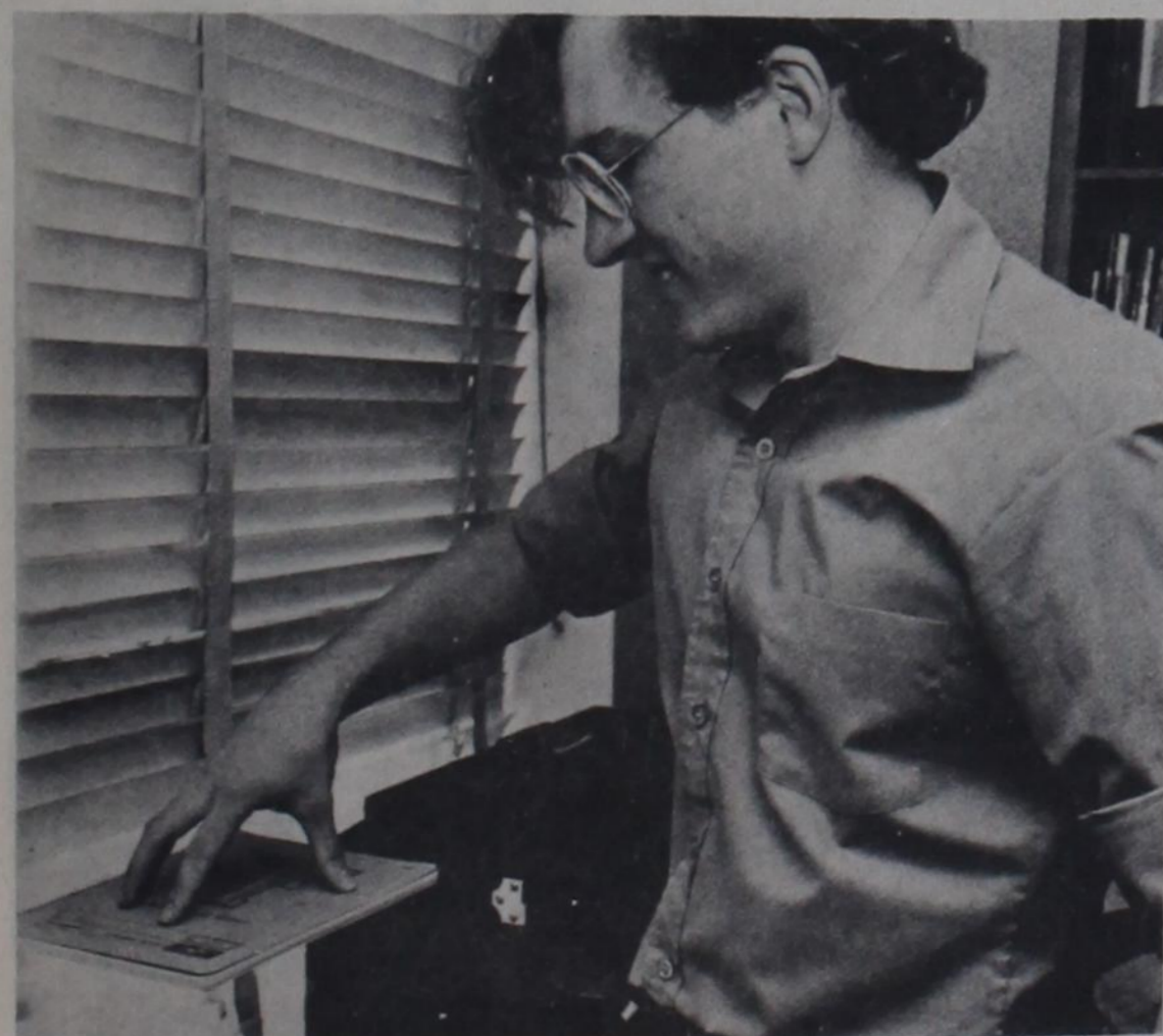
NO GIMMICK — Gary Gimble shows how forceful the air is coming out of the wall ventilators in Murdough Hall.
