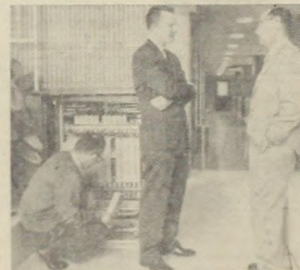
"4:10 P.M. At the Port of Galveston offices, I discuss advantages of the new P.B.X. with one of the officers of the Port. The Port requires complex telephone services, which must be maintained around the clock."
