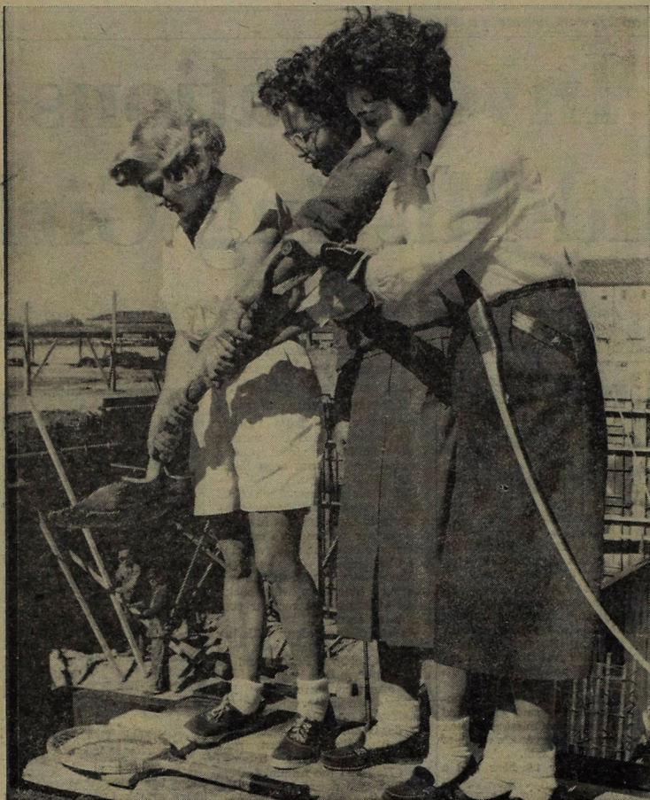
THREE PRETTY TECHSANS TAKE A HAND AT WORK ON NEW WOMEN'S GYM . . . contractors look on in anguish as girls decide to hurry construction
