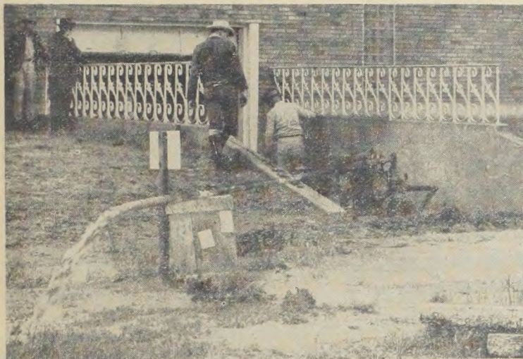
ALL WET—Lubbock residents weren't the only ones bothered by flooding during the recent downpour. Tech also got its share, as indicated by the picture above. Workmen, directed by George Long, superintendent of buildings and grounds, pump water from the basement of the Library building. Flooding was only partial, covering the shipping room and a portion of the stacks. Resulting damage was slight. (Photo, Margaret Allen.)
