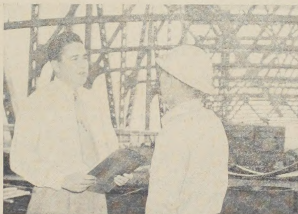
Bill Rhode (left) at the site of New Orleans' new Claiborne Street Industrial Canal Bridge.
