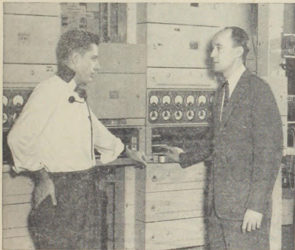
Dick Walsh (right) discussing carrier equipment which will provide many additional long distance circuits out of Philadelphia.
