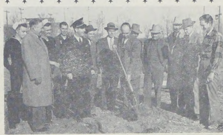
NAVAL RESERVE ARMORY CONSTRUCTION STARTED—Pres. W. M. Whyburn, center, wielding the shovel, presided at informal ground-breaking ceremonies Tuesday morning for the $127,780 Naval Reserve armory to be constructed southeast of the old football stadium.
