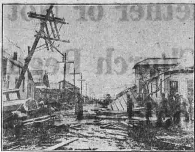
Here are two views of damage done by the wind of tornadoic force which dipped into lower New Orleans, demolishing or damaging about 100 homes and seriously injuring at least 12 persons. (Associated Press Photo)
