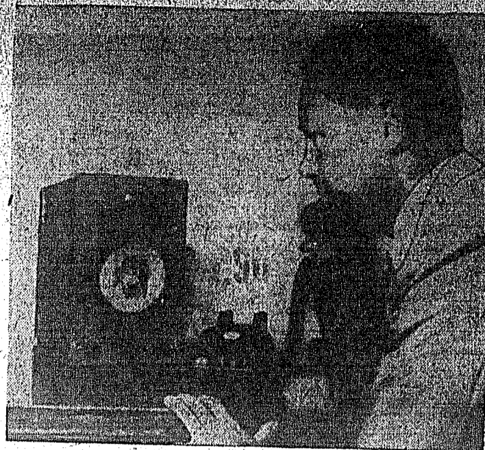
PICTURE PHONE . . . Bell Telephone Laboratories exhibits telephone transmitting photos with sound. Camera lens is above 2x3 inch picture.
