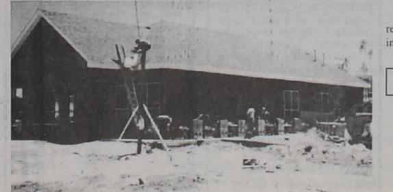
CONSTRUCTION CONTINUING - The construction continues on the Gorman Post Office. Brick is now being laid this week. The inside construction continues also. Window Frames are in place
