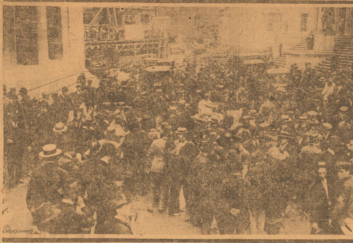
Crowd before Morgan bank after explosion seeking friends and relatives. At right is the sub-treasury building.
