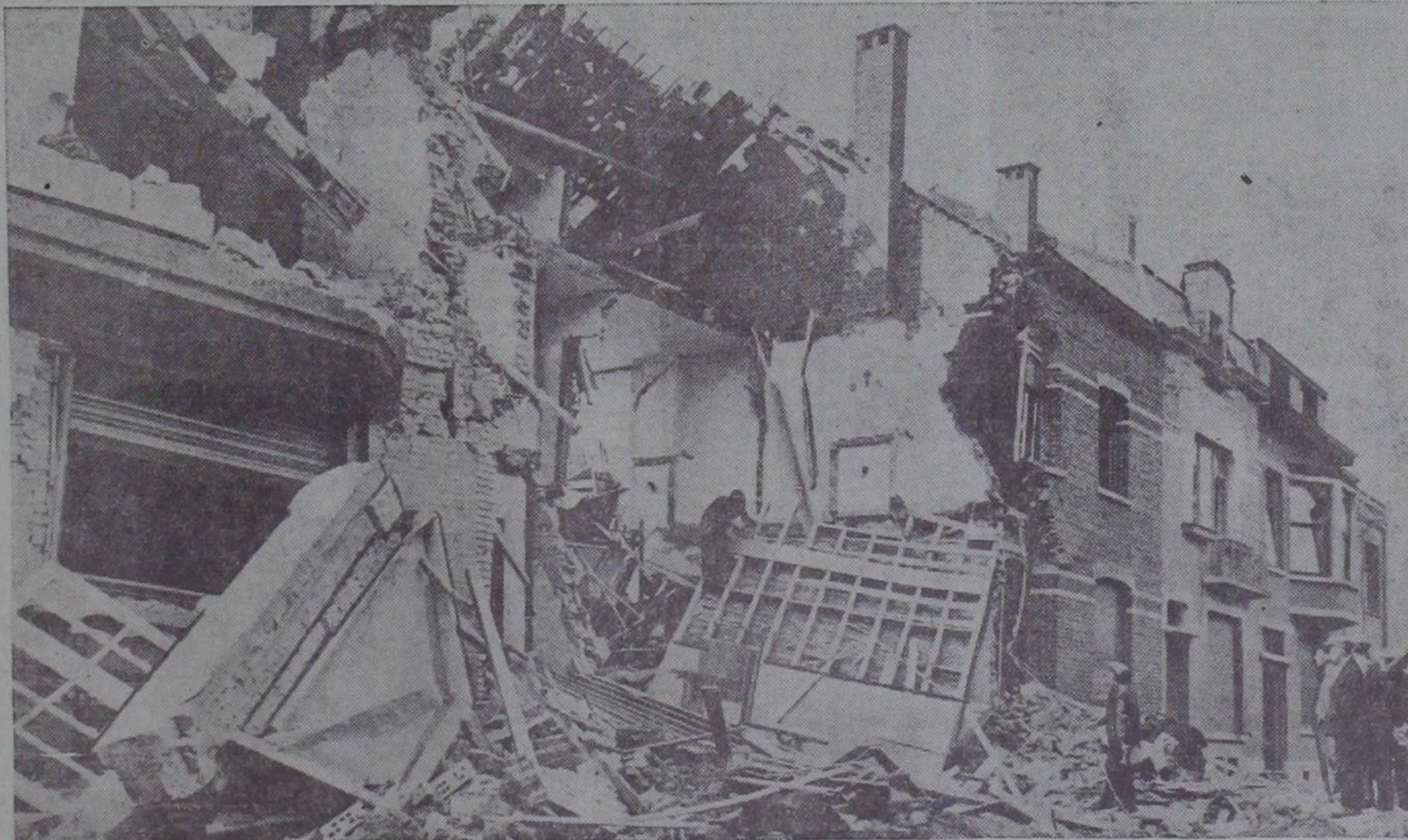
MORE AND MORE frequent in France are such scenes as this one, with intensification of aerial warfare. Towns and cities are suffering more and more from accurate bombing on the part of the Germans and the Allies. This particular wreckage was photographed at Nancy, in Northeastern France.
