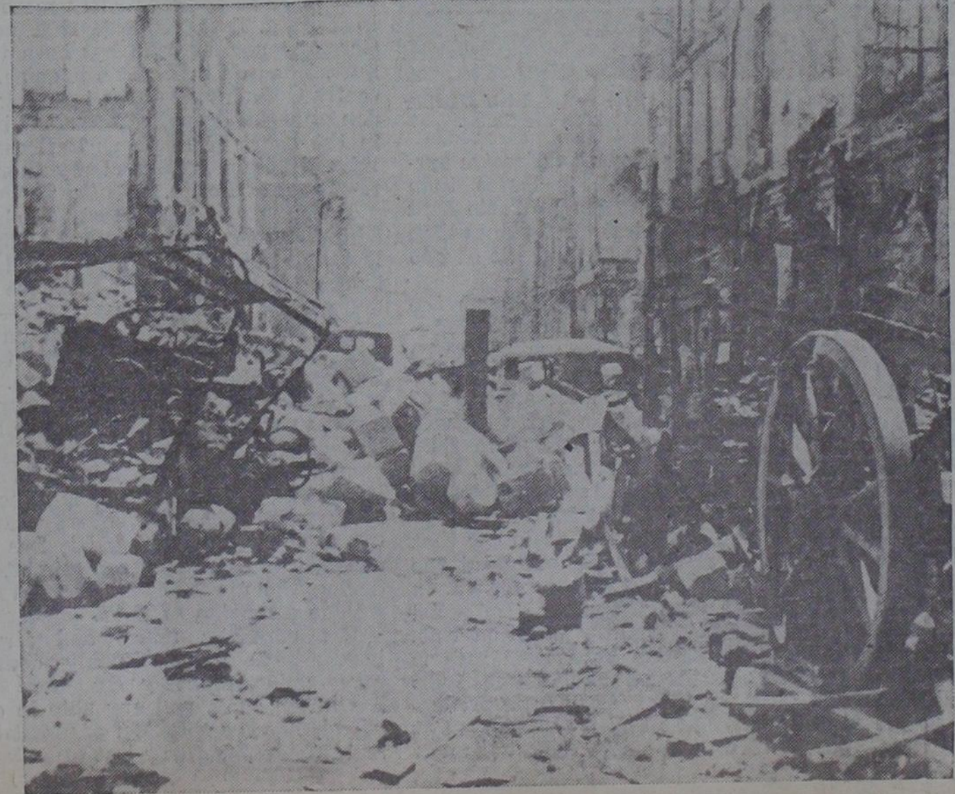
ROAD CLOSED —A street in Orleans, France, literally choked with debris, shows terrific blasting given town by Nazis' huge bombers.
