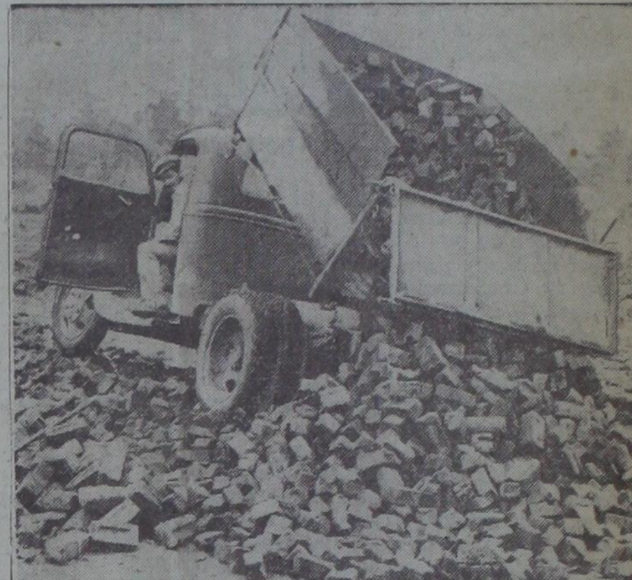
LONDON TO HOUSTON —Brought to this country as ballast aboard a British freighter, bricks from bomb-torn London become part of Houston, Texas, highway. They'll serve as road foundation.
