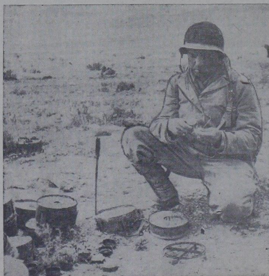
TAKING OUT THE STING —This is how U. S. Engineers removed detonators from mines taken from shoulders of road during battle for Big Barbott Pass, Tunisia. Americans won pass and pushed Axis toward Gabes.
